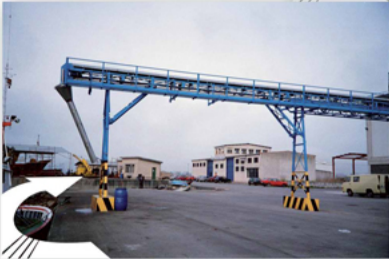
Equipment TTL with walkway, covering and chute of unloading with pipe.
