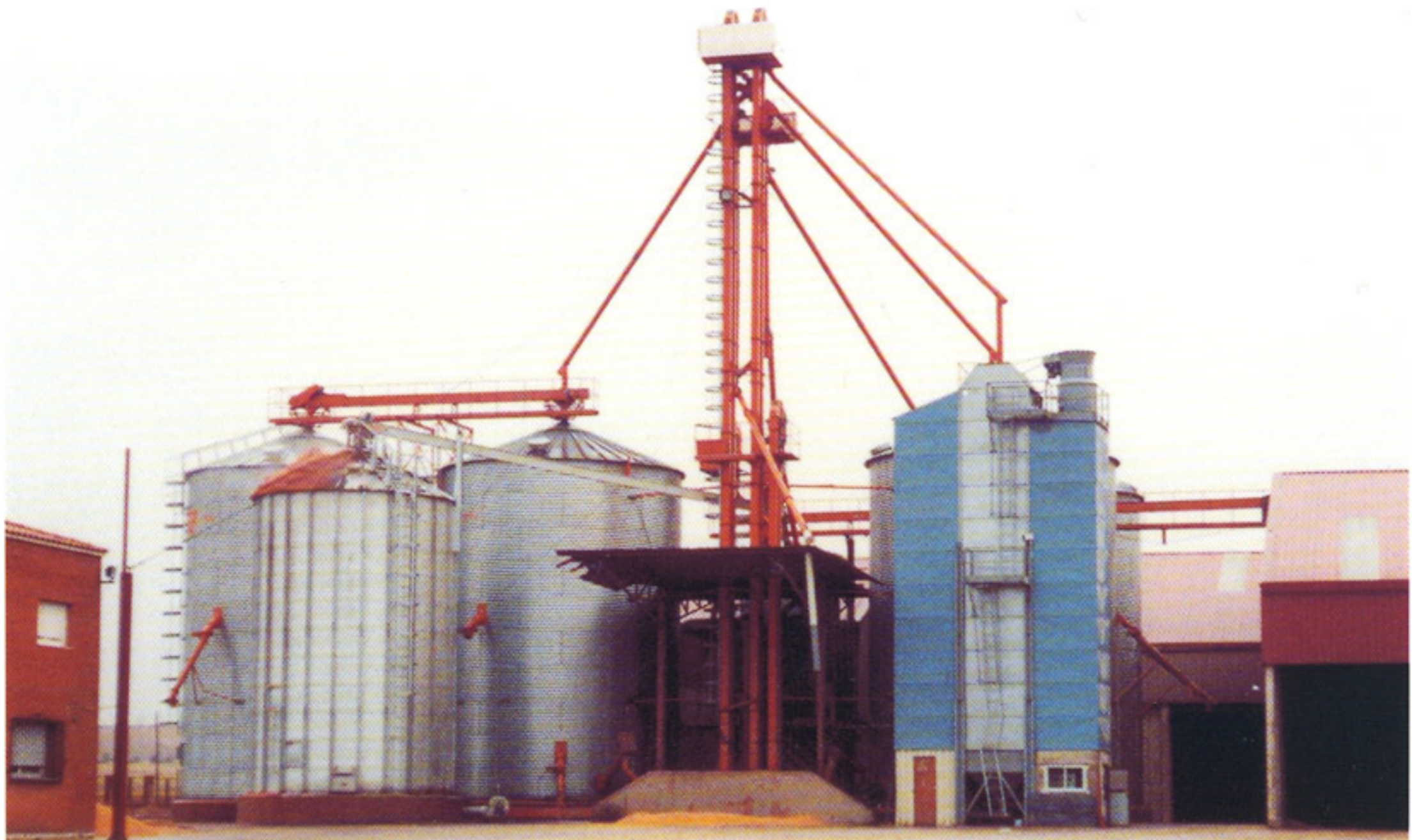
TEC installation for agricultural sector.
