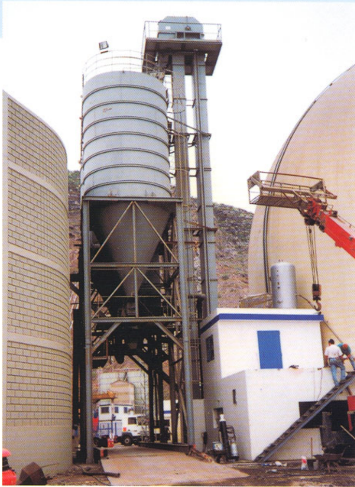
TEC installation for concrete storage in bin.
