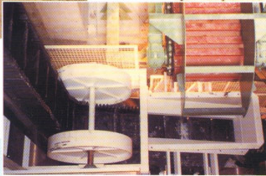
Detail of loading header.
