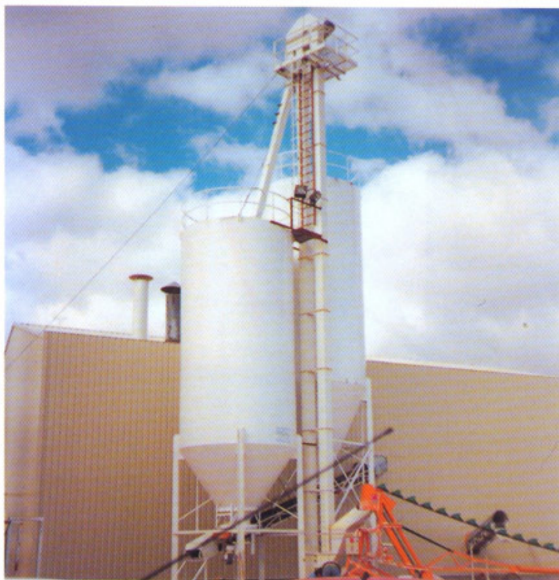
TEC conveyor for dispenser installation.
