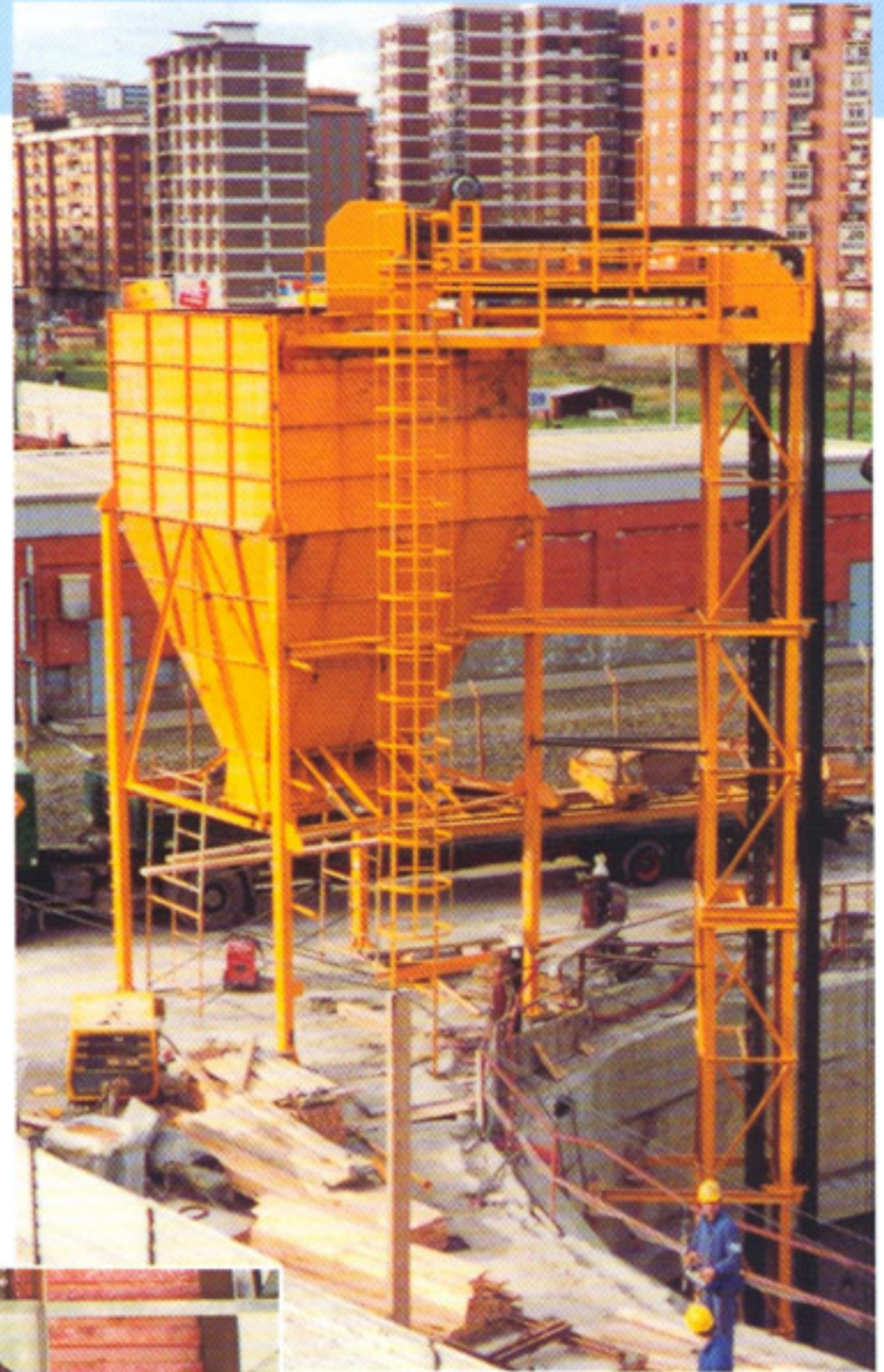
TEB for extraction from 33 m. profundity of excavation in the collector tunnel, with hopper and truck loading system.
