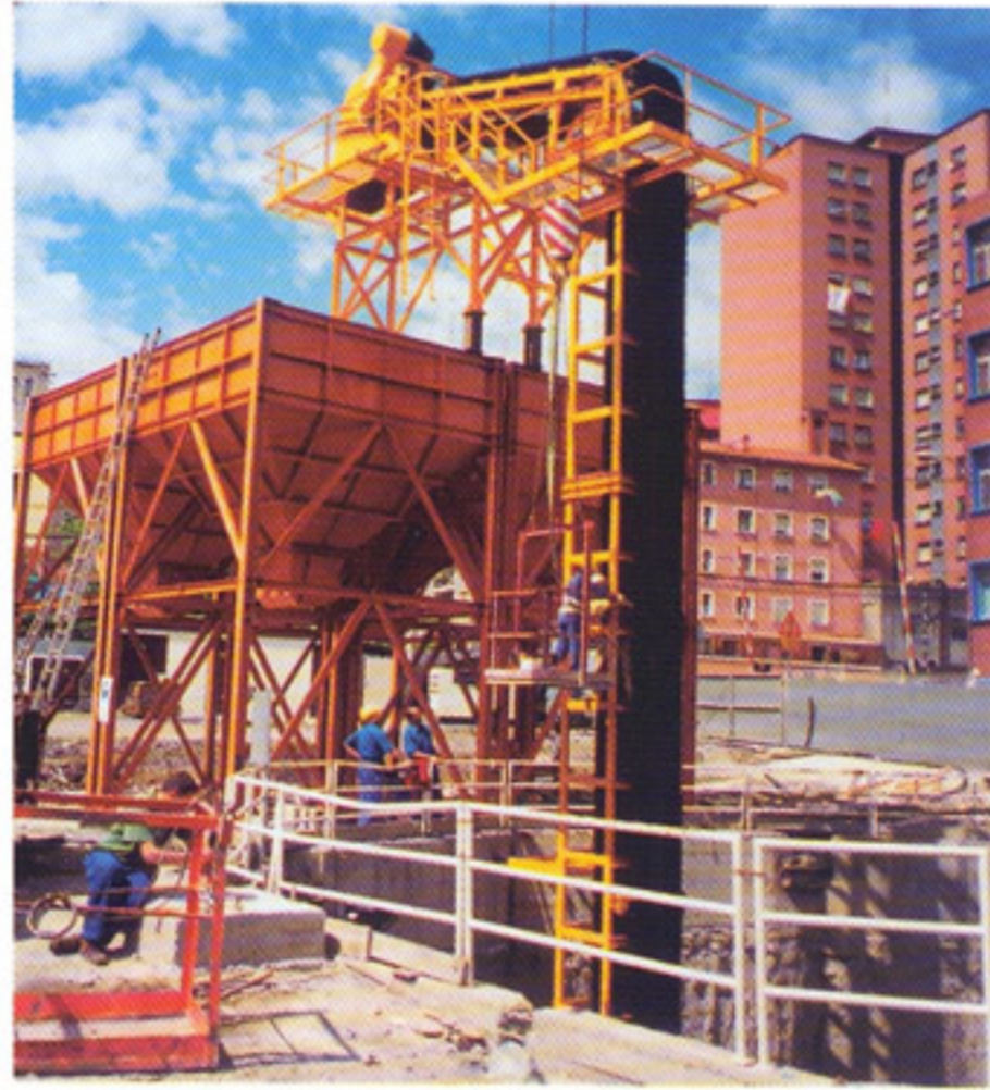
TEB conveyor installation for digging.
